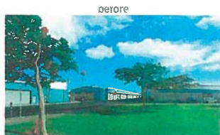
Cooke Street and Mother Waldron Park These Kaka'ako warehouses are what Eric Crispin, AIA, the city's director of planning and permitting, calls a "remnant land use." Their existence dates back to a time when a separate warehouse district was needed to supply the nearby Honolulu business district. Mother Waldron Park provides some pleasant, if pointless, green relief—it's a neighborhood park without a neighborhood. (The park's name is credited to Kaka'ako historian, named after the area's original inhabitants.)
