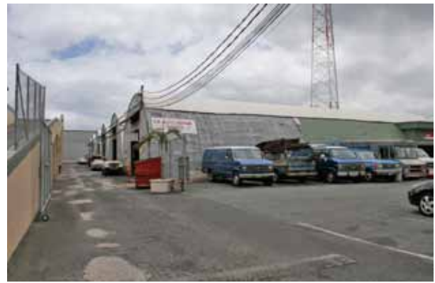
Figure 5-16 Six Quonset Huts
