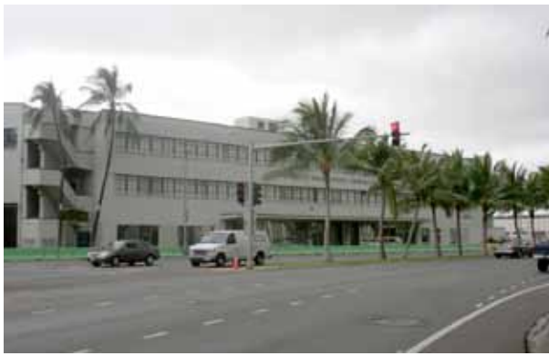
Figure 5-57 DOT Harbors Division Building
