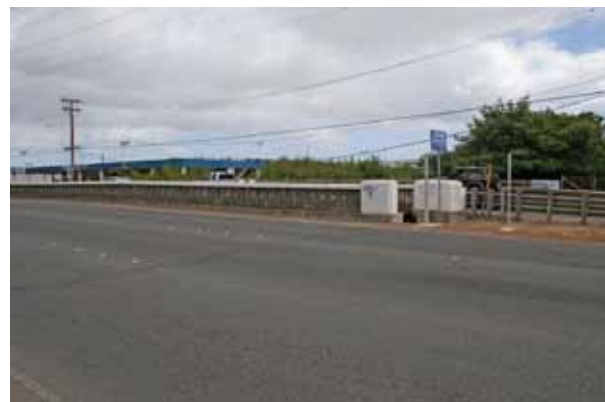
Figure 5-44 Waimalu Stream Bridge
