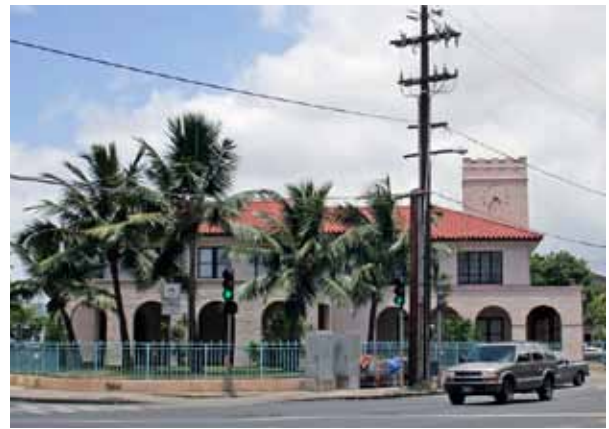
Figure 5-18 O'ahu Railway & Land Company Terminal Building
