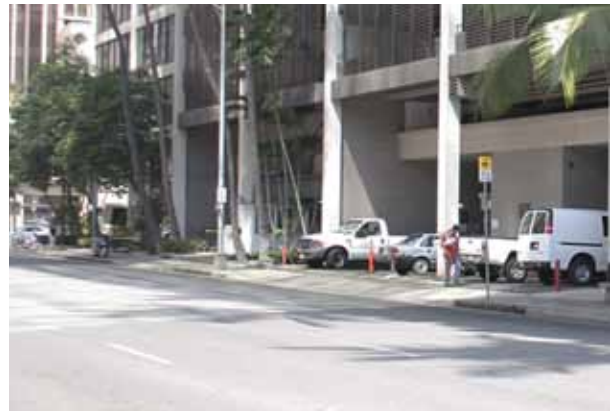
Figure 5-30 Parking Entrance at Harbor Square Building
