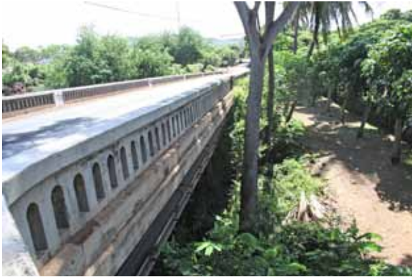
Figure 5-43 Waiawa Stream Bridge
