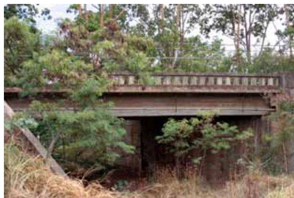
Figure 5-41 Honouliuli Stream Bridge
