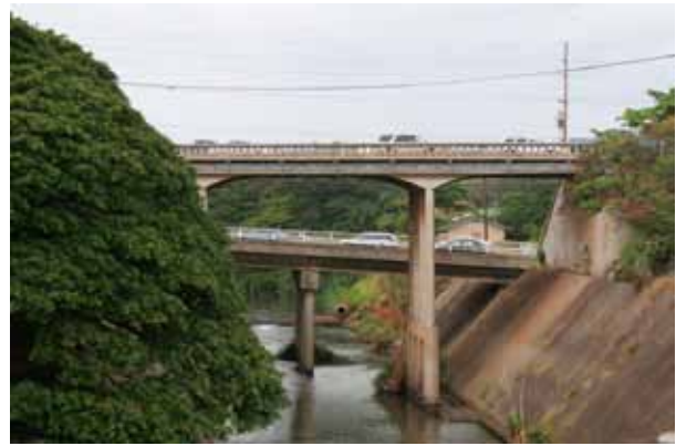
Figure 5-42 Waikele Stream Bridge, Koko Head Span
