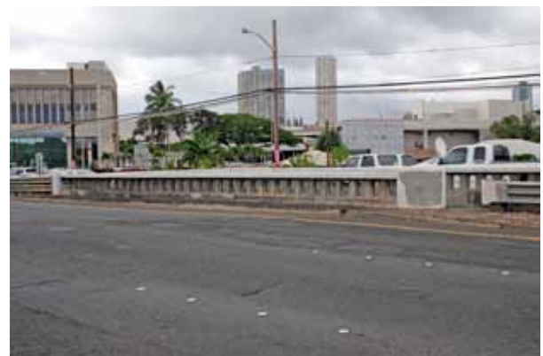
Figure 5-46 Kalauao Stream Bridge
