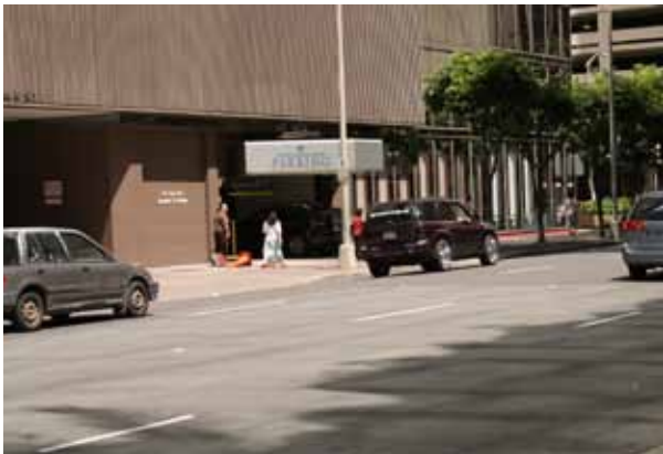
Figure 5-29 Entrance to Pacific Guardian Center
