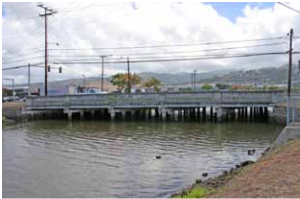
Figure 5-15 Kapālama Canal Bridge
