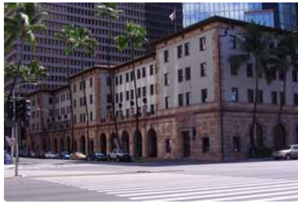
Figure 5-25 Dillingham Transportation Building, looking Mauka from Nimitz Highway
