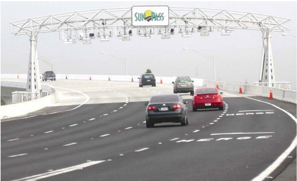
Figure C1. A single gantry facilitates tolling both directions of REL.
