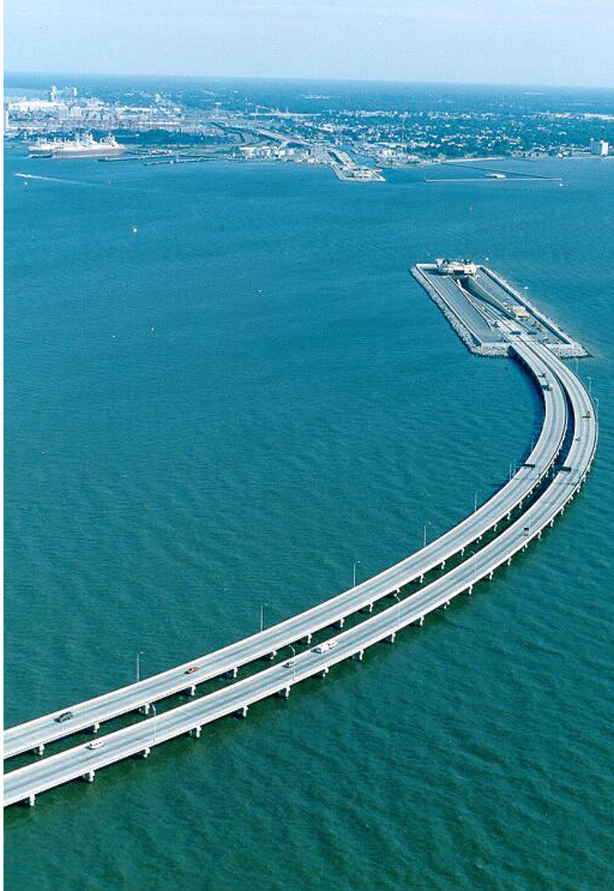
Figure 6.4. Monitor-Merrimac Memorial Bridge-Tunnel (I-664), looking north. Starting at the left edge of the photo is the Newport News U.S. Marines Terminal.
