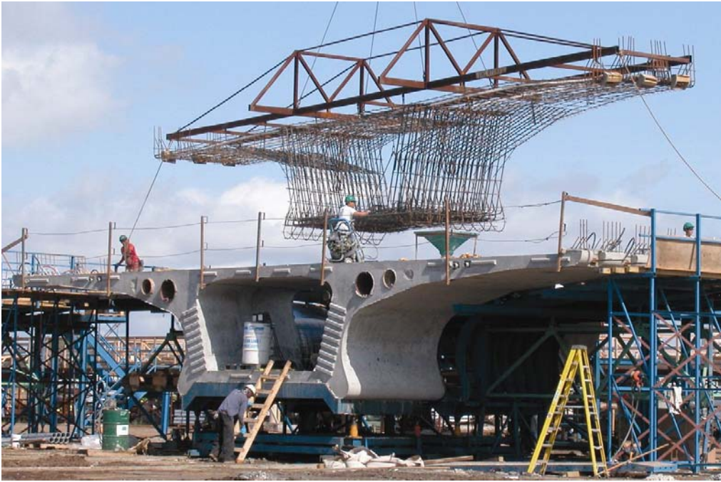
Figure C2. The segmental yard cast-matching technique was responsible for excellent on-site fit and large economies in construction.
