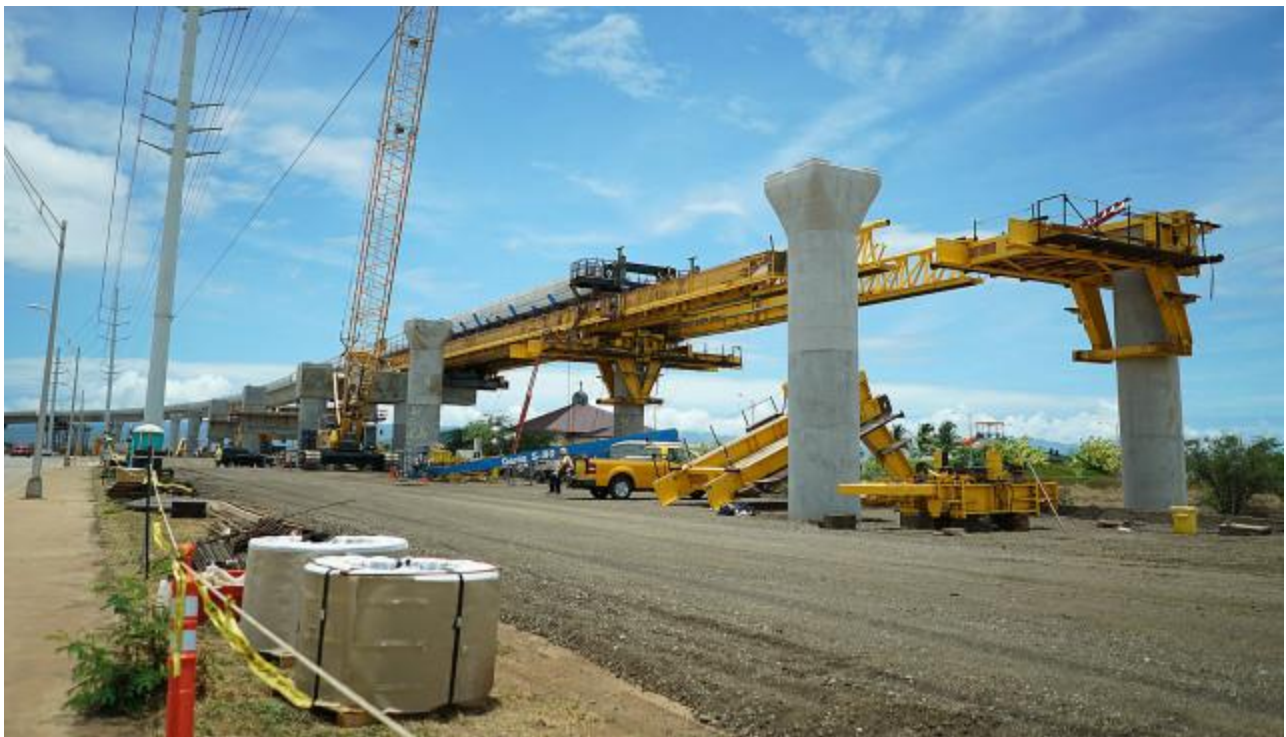
The rail guideway as it took shape in 2015 along Kualakai Parkway in Kapolei.
